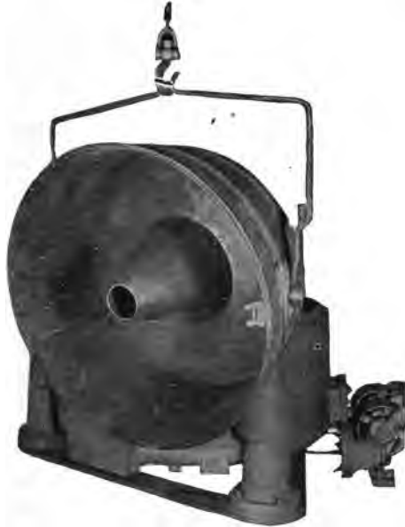
FIG. 38.—Inverted Basket of Centrifugal Machine.
